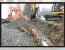
the Greenshores guidelines. Beach nourishment is the process of adding new sand, gravel and/or cobble to a beach. This doesn't stop erosion but the new material gives the waves something to erode. Large logs were placed at the bottom of the eroded slope and along the top of the beach. These logs help keep the new sand and gravel in place, break waves as
